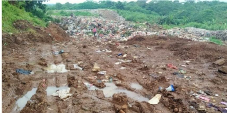
Figure 1. TPA Bangkonol Operational Road Conditions
