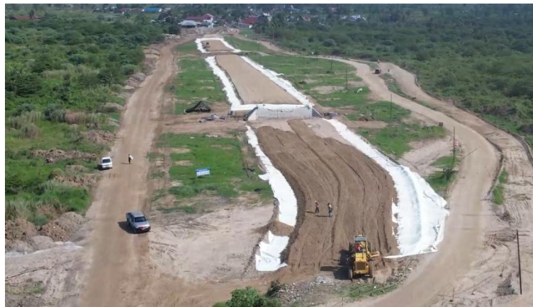
Figure 8. Implemented rehabilitation and reconstruction
