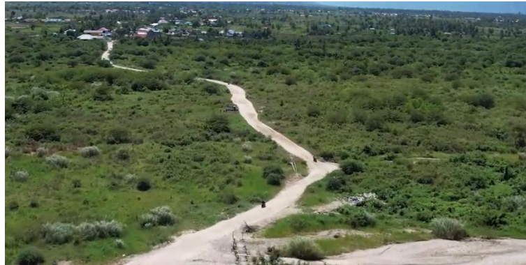
Figure 3. Road geometric condition in January 2022
