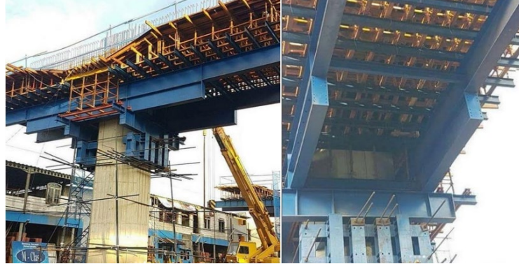
Figure 1. Cantilever system formwork on the pier-head of the Becakayu Toll Road
