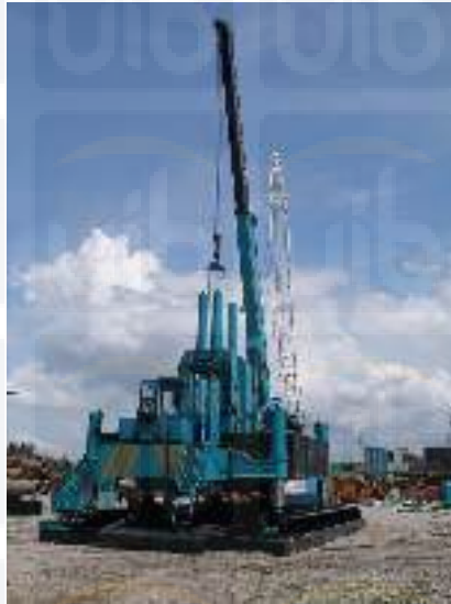
Gambar 2.13 : Jack In Pile
