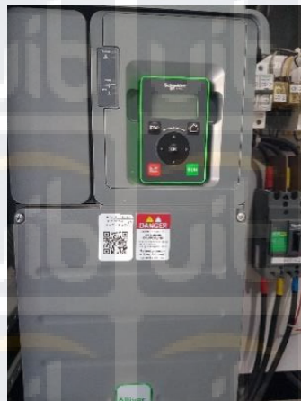
Gambar 2.6 VSD Schneider ( Illustration only )
