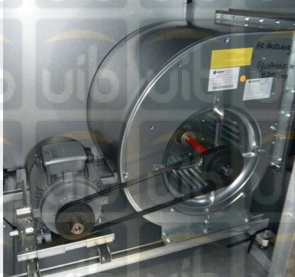
Gambar 2.4 Blower fan dan motor ( Illustration Only )
