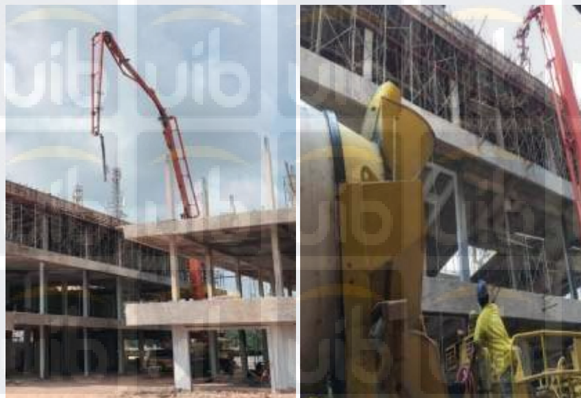
Gambar 4.1 : Concrete Pump dan Molen Readymix
