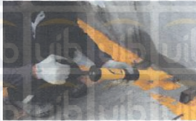
Gambar 4.14. Pemberian Joint Bonding
