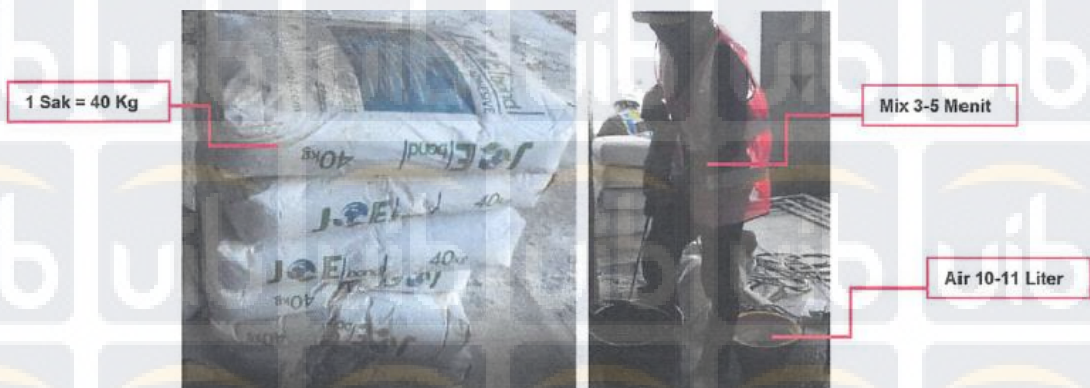
Gambar 4.9. Pencampuran Joint Bonding
