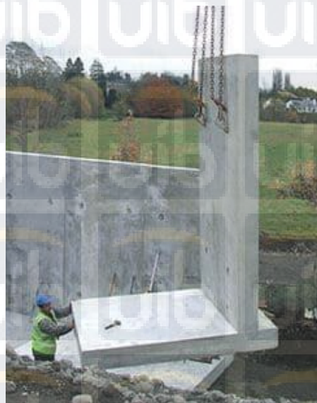
Gambar 2.5. Cantilever Retaining Wall
