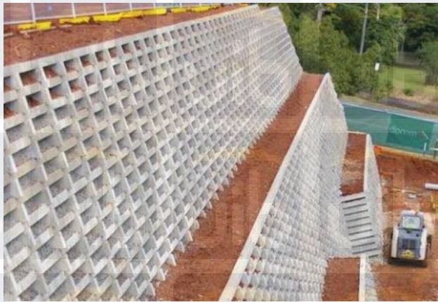
Gambar 2.3. Crib Retaining Wall
