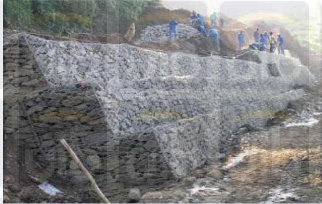
Gambar 2.4. Gabion Retaining Wall
