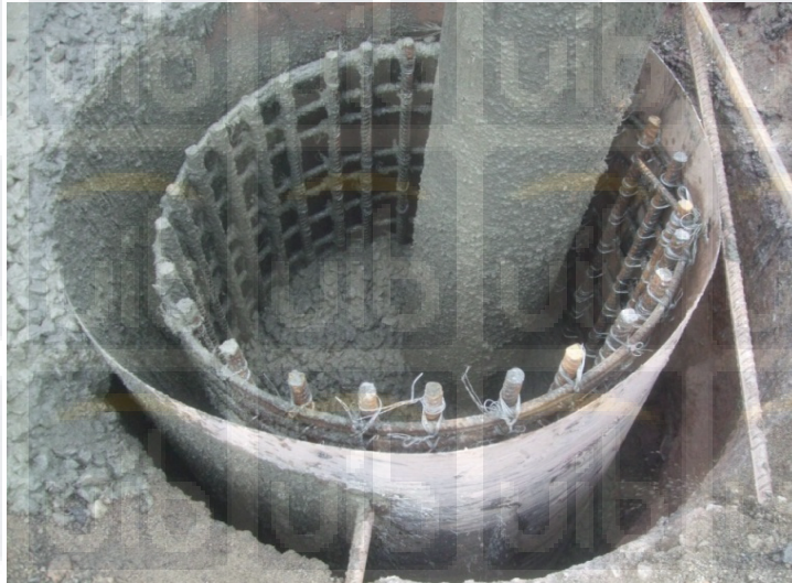
Gambar 4.2 Proses Pondasi Bored Piled
