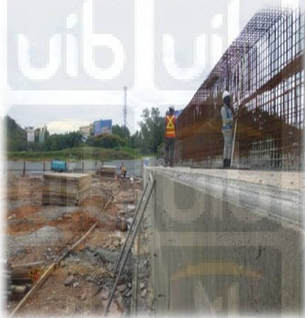
Gambar 4.18 Proses Pengerjaan Abutment
