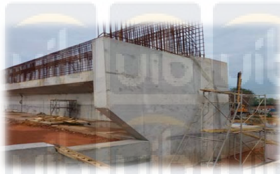
Gambar 4.18 Proses Pengerjaan Abutment
