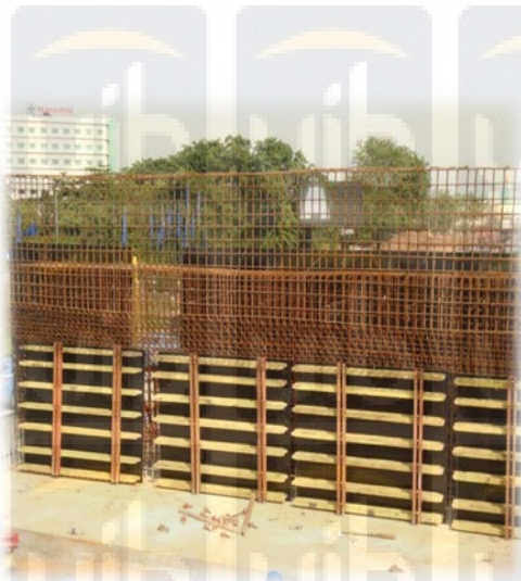
Gambar 4.18 Proses Pengerjaan Abutment
