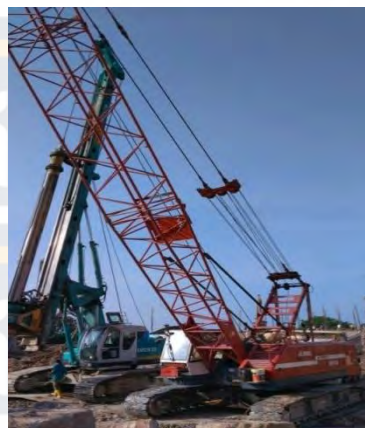
Gambar 4.3 Crane Services Fuwa QUY 55
