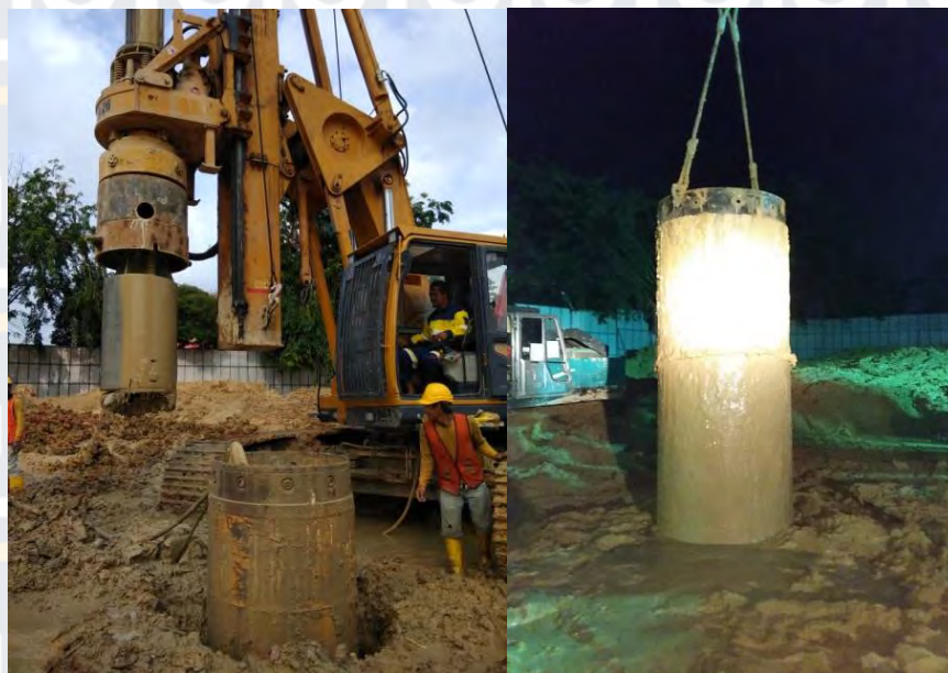
Gambar 4.7 Casing Driver
