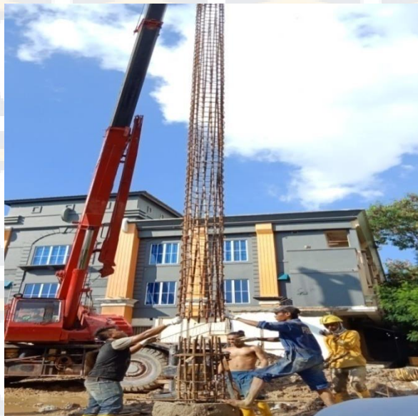
Gambar 4.6 Setting tulangan besi
