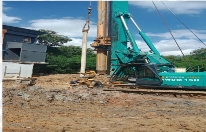
Gambar 4.7 Setting pipa tremi
